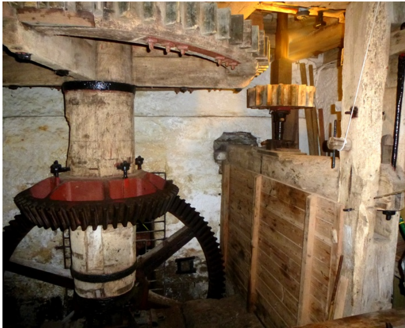
Figure 13: The pit wheel, wallower, upright shaft, great spur wheel and one of the stone nut gears at Stretton water mill, Malpas, Cheshire.
