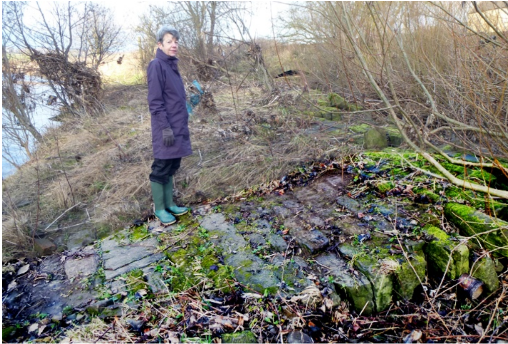
Figure 10: Large cobble stones set in the earth bank upstream of the arch. They slope gently towards the river at an angle measured as 11^\circ .
