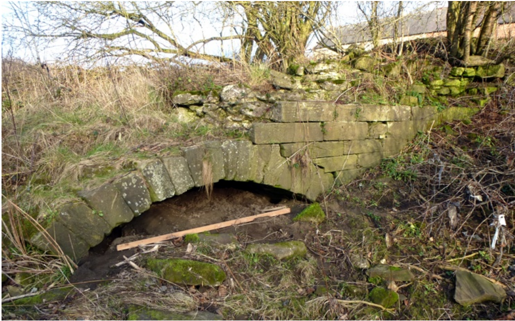
Figure 8: The silted up mill arch in February 2017. The wooden stick is 68 inches (172 cm) long.
